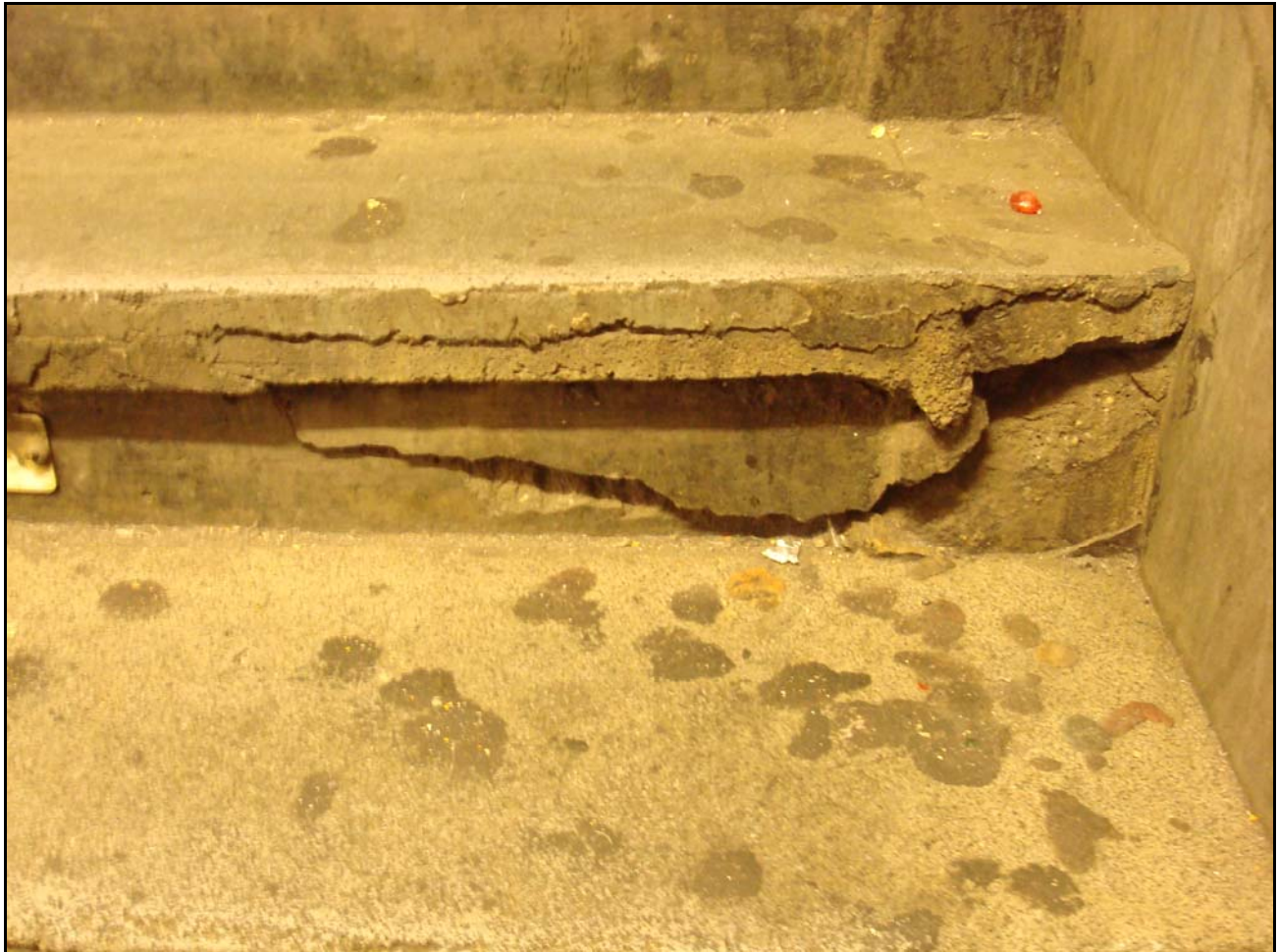
149 th Street Grand Concourse
