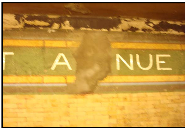
138 th Street Grand Concourse
